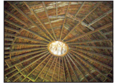
The beautiful skeletal structure of the roof
