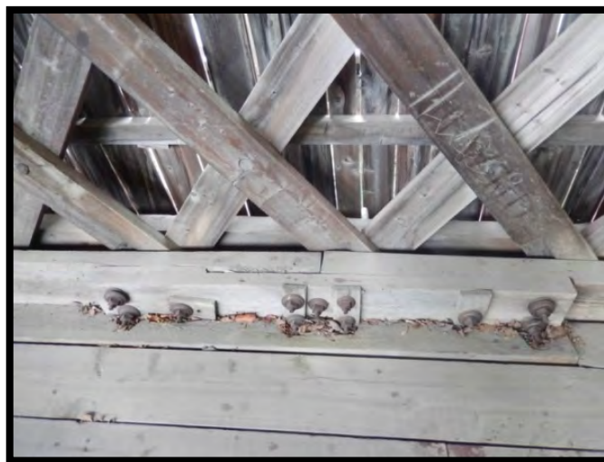
Photo No. 10 – Truss and reinforced spliced joint Michael Grayson
