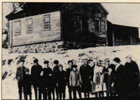
Cooledge School Knowlton's Landing
