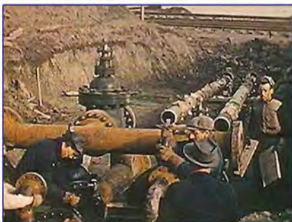
Montreal Pipeline - Construction
